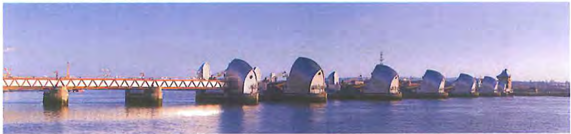
Figure 1 Thames Barrier, London
