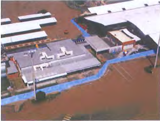
Demountable levee round Rockhampton Airport (2011)
