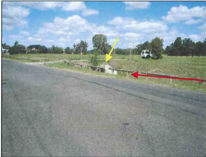
Photo 1: View looking southwest over the site from North Street. Note the existing culvert pipe and crossing that provides access to the site (refer yellow arrow) and the swale drain located along the site frontage (refer red arrow).
