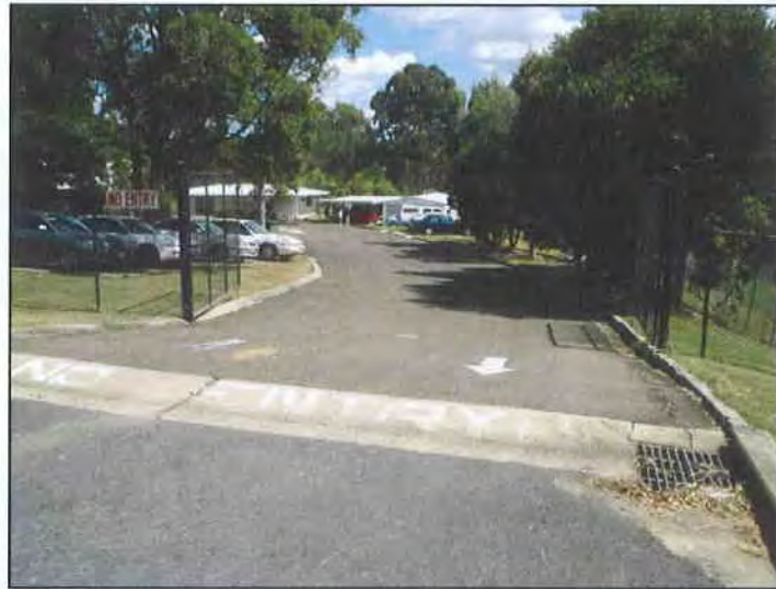
Photo 7: A Queensland Transport service centre adjoins the sites southern boundary and gains access via Colvin Street.
