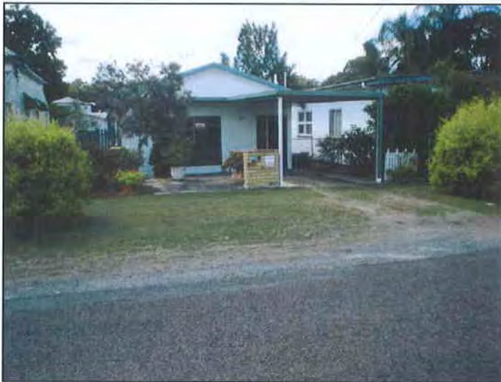
Photo 5: Established residential properties are located to the east of the site on the opposite side of North Street. These dwellings are typically constructed of timber cladding with corrugated iron roofs and utilise a variety of colours and roof pitches.
