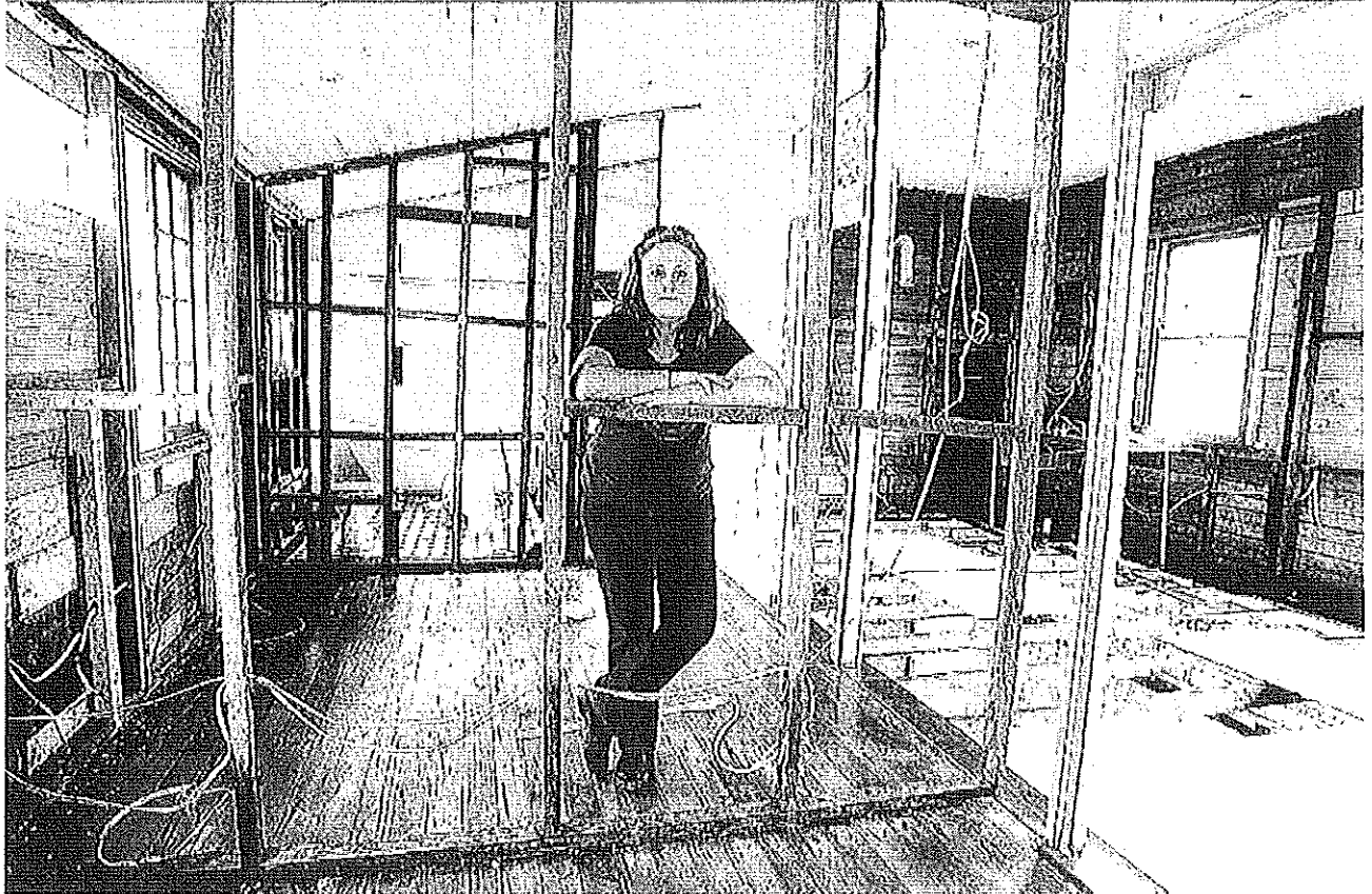
TRAUMATIC DAMAGE: Social worker Sally Doyle surveys the damage at her flood-wrecked West End home
