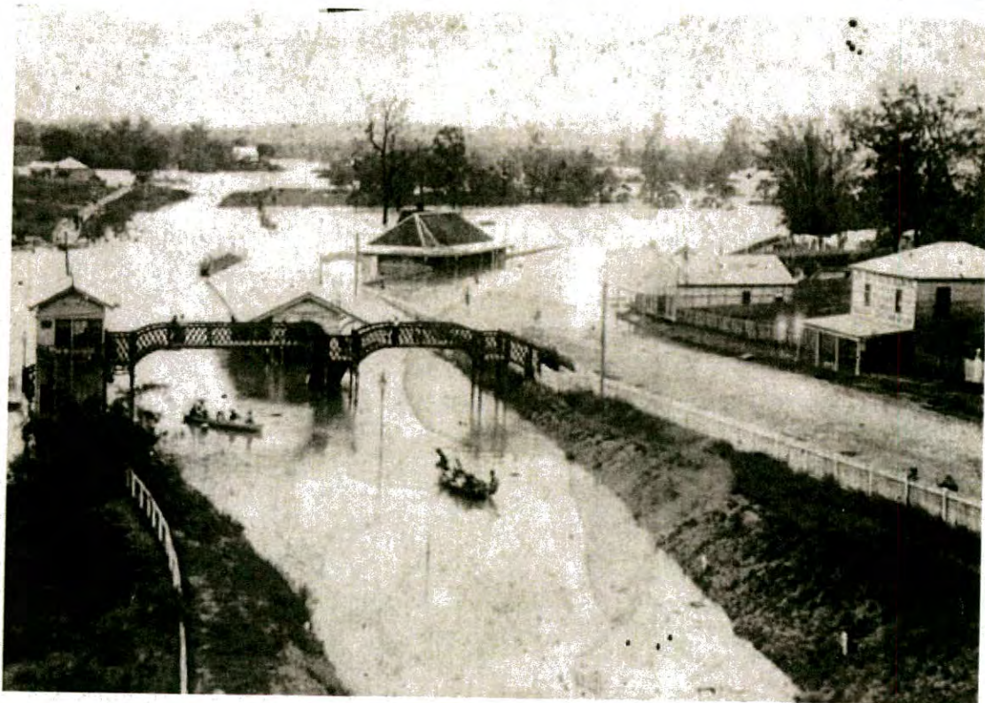
Toowong Railway Station during 1893 flood
