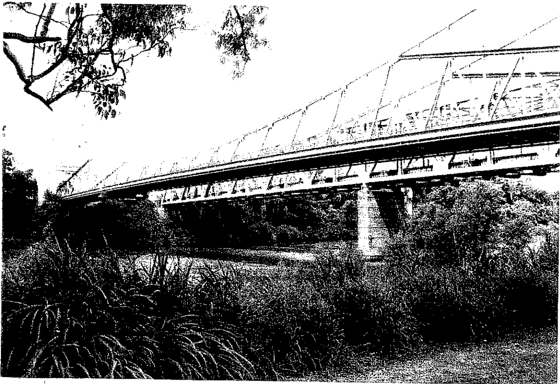
STRUCTURE 2-INDOOROPILLY BRIDGES (LOOKING DOWNSTREAM)
