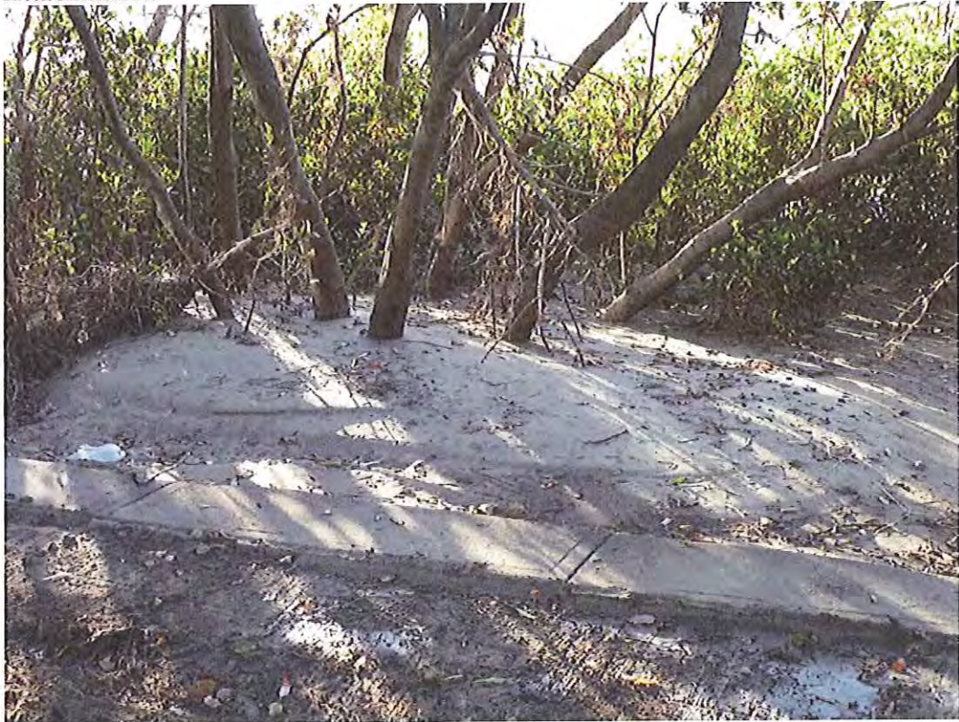
Figure 1: Mud and sand deposited amongst mangroves, Riverside Drive, West End
