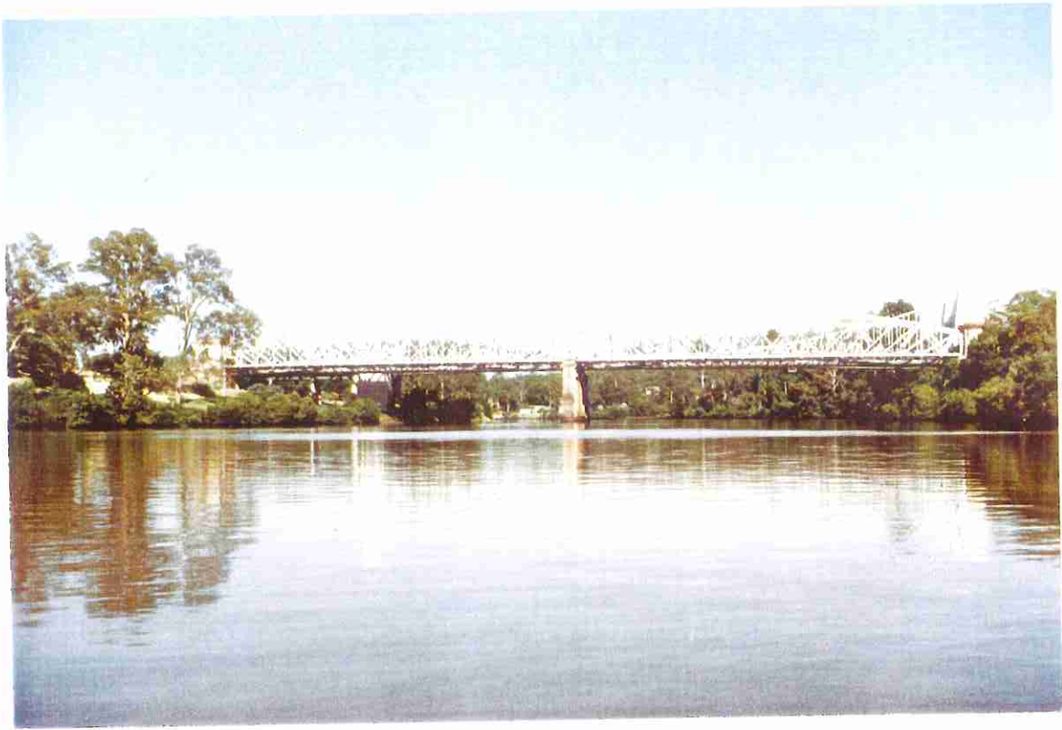
STRUCTURE 2-INDOOROOPILLY BRIDGES (LOOKING UPSTREAM)
