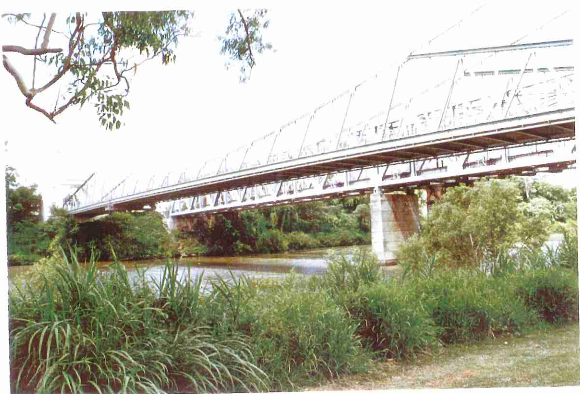
STRUCTURE 2-INDOOROOPILLY BRIDGES (LOOKING DOWNSTREAM)
