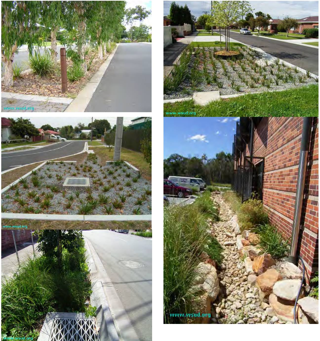
Figure 9.1 Optional Configuration of Bioretention Systems (source: www.wsud.org )
