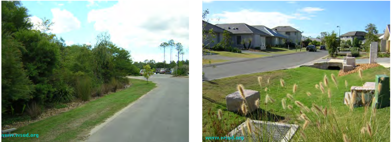
Figure 9.4 Example Applications of Swales (source: www.wsud.org )
