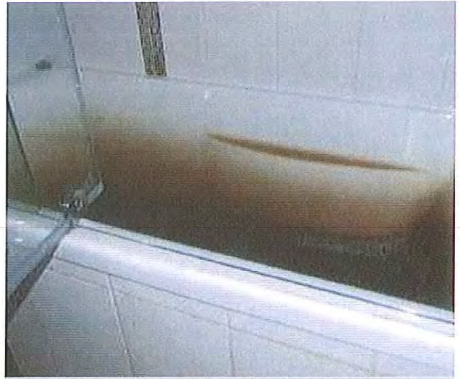
13/01/2011, 10:06:06 am: Showing muddy water that came up through the bath plumbing but did not overtop the bath
