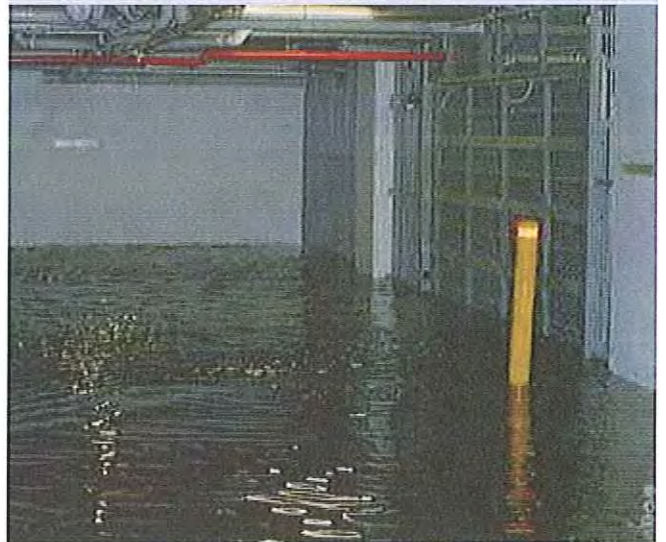
12/01/2011, 7:16:47 am: Aura gate entrance to carpark in basement 1
