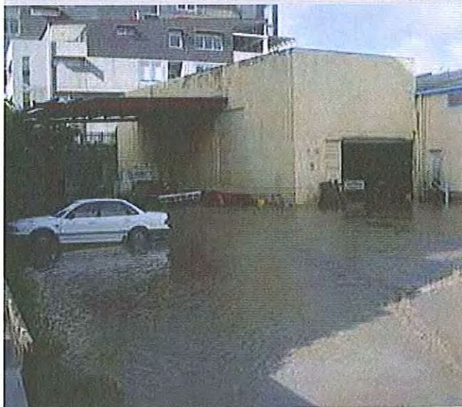
12/01/2011, 7:47:15 am: Water entering the construction business next door to Aura on the western side
