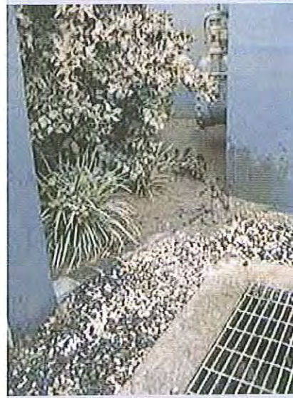
14/01/2011, 2:44:30 pm: Stormwater surged up through this drain, pushing the mud aside
