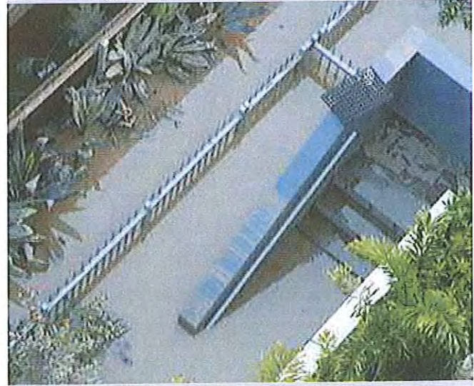
13/01/2011, 5:14:18 pm: Looking down to Aura's back entrance and sunken garden showing flood line and water receding
