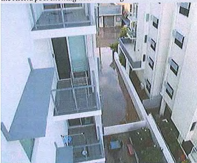
13/01/2011, 5:13:12 pm: View showing water still covering the entrance to the Aura basement carparks
