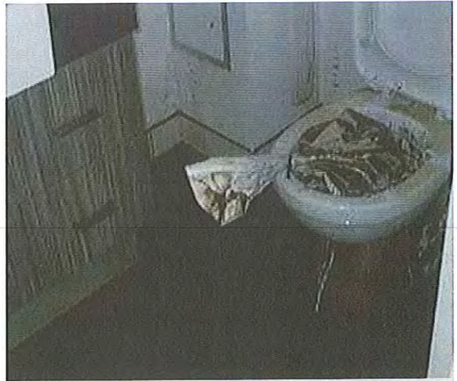
13/01/2011, 4:00:44 pm: Showing flood level on pedestal and muddy water coming up inside toilet bowl in Unit [redacted], Aura
