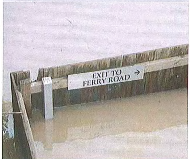
13/01/2011, 10:48:44 am: Looking down to the back corner fence of the Aura property on the western side
