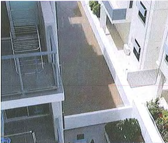
12/01/2011, 1:19:23 pm: Looking down on to the Aura carpark entrance
