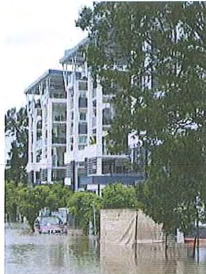
13/01/2011, 12:45:46 pm: View from river end of Ferry Road showing the flooded red car in front of Aura Apartments
