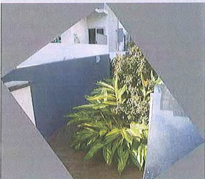
12/01/2011, 7:47:05 am: Water entering the sunken garden surrounding Aura
