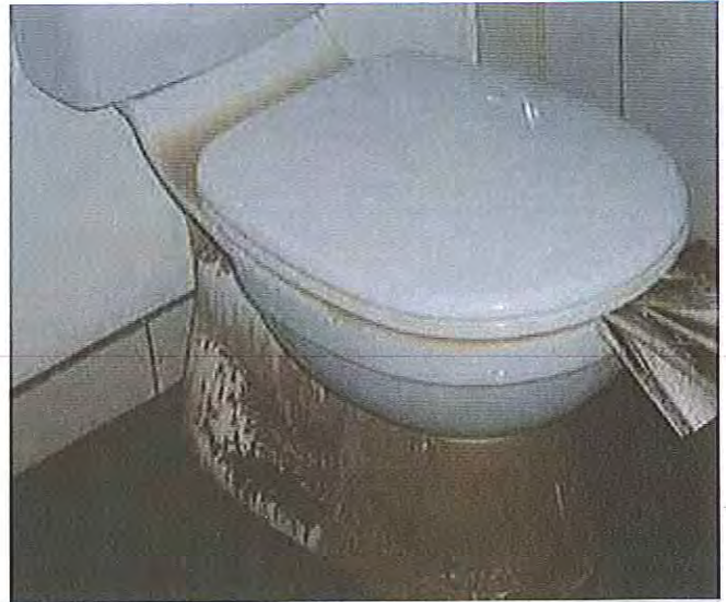
14/01/2011, 12:33:50 pm: Toilet (Unit 4, Aura) showing flood level on pedestal and muddy water coming up into toilet bowel
