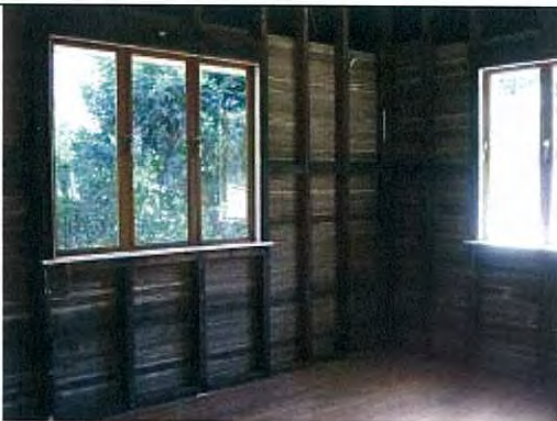
Photo #5 : Interior Walls
