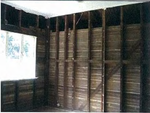
Photo #3 : Interior Walls
