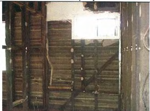
Photo #4 : Interior Walls
