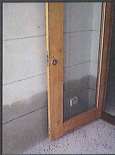
High water mark on blockwork
