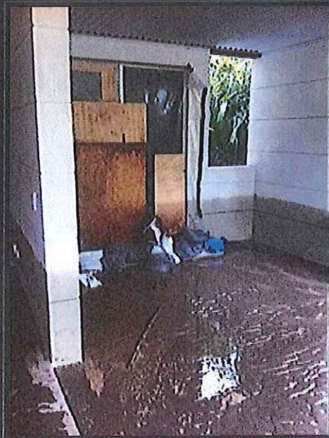
Door to lower hallway, protected with ply, plastic and sandbags
