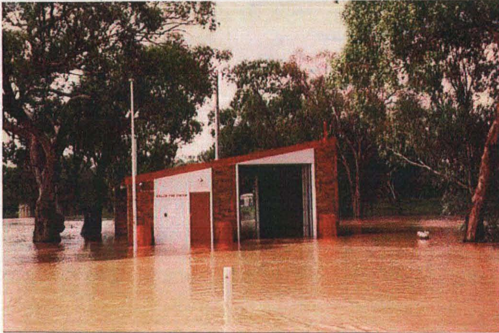
Plate 6: Bollon fire station during the 1997 flood (Max Henderson photo)
