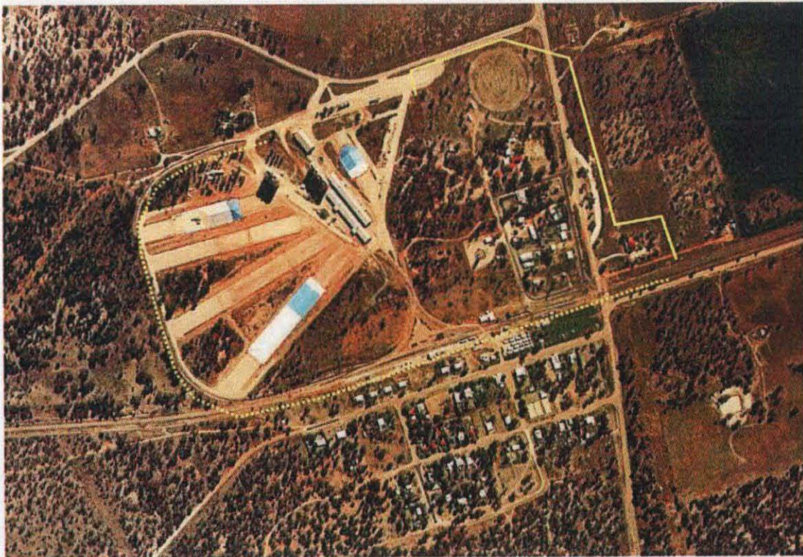
Plate 2: Thallon levee and railway embankments (BSC photo – 19 September 1999)
