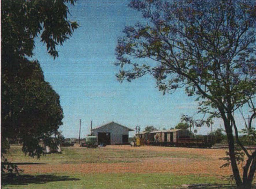
Plate 15: Rail freight facility at Dirranbandi
