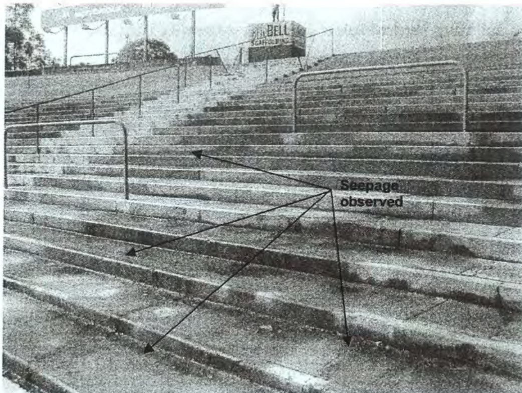
Figure 5.7.1 Ground Water Seepage At Southern Outer
