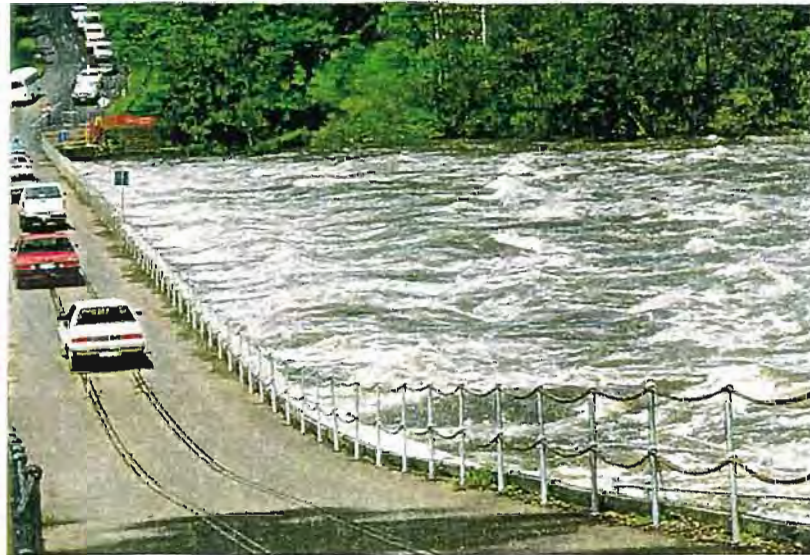
Figure 12.3 & 12.4 Mt Crosby Weir Bridge – 1400 hrs Friday 12 th February Fernvale Bridge, with an immunity of approximately 2000 m 3 /sec remained opened at all times during the event with a small clearance between the underside of the bridge beams and the flow. This clearance was less than 200 mm at times.
