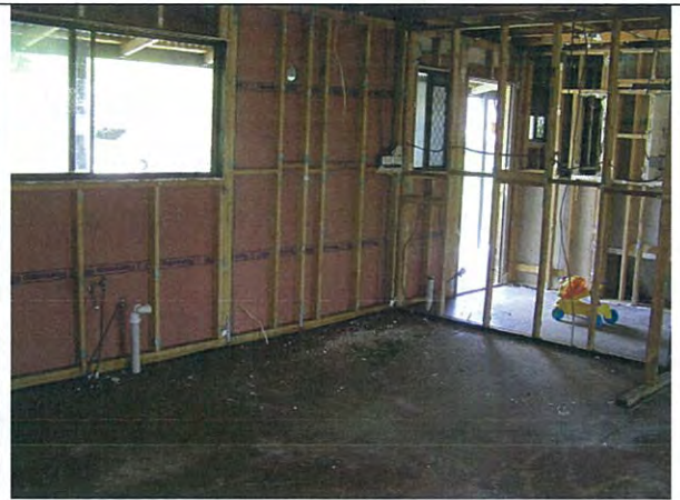
Photograph 2 – gyprock stripped out
