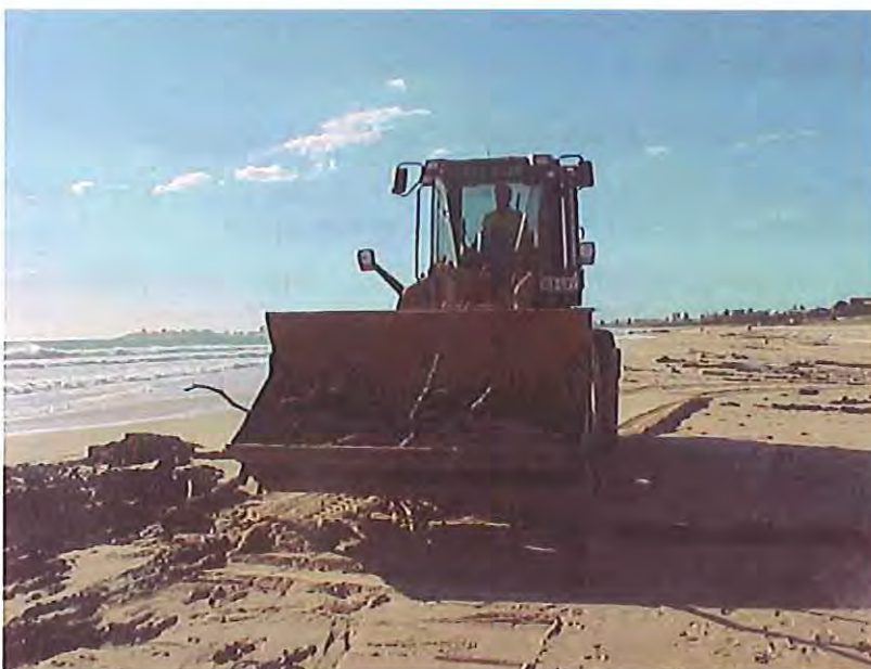
Beach debris clearing, 2004 following flooding and storms
