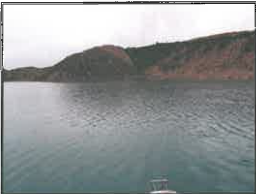
Figure A1.3: Heavily eroded banks
