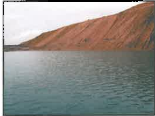
Figure A1.2: High spoil bank
