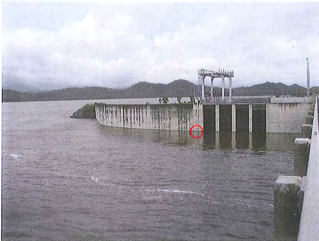
This picture above was taken at 5.42pm 10 th January 2011. At this time, the automatic headwater gauge (ALERT Id 6637) was reading 72.91m and the staff gauge reading was 72.92m AHD. Note the laminar nature of the flow around the stilling well and the lack of turbulence. At the time, the outflow was the dam was 2,400m 3 /s.
