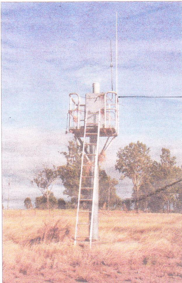
■ VITAL EQUIPMENT: One of the 38 new river gauging systems the CHRC has installed since the 2008 floods.
