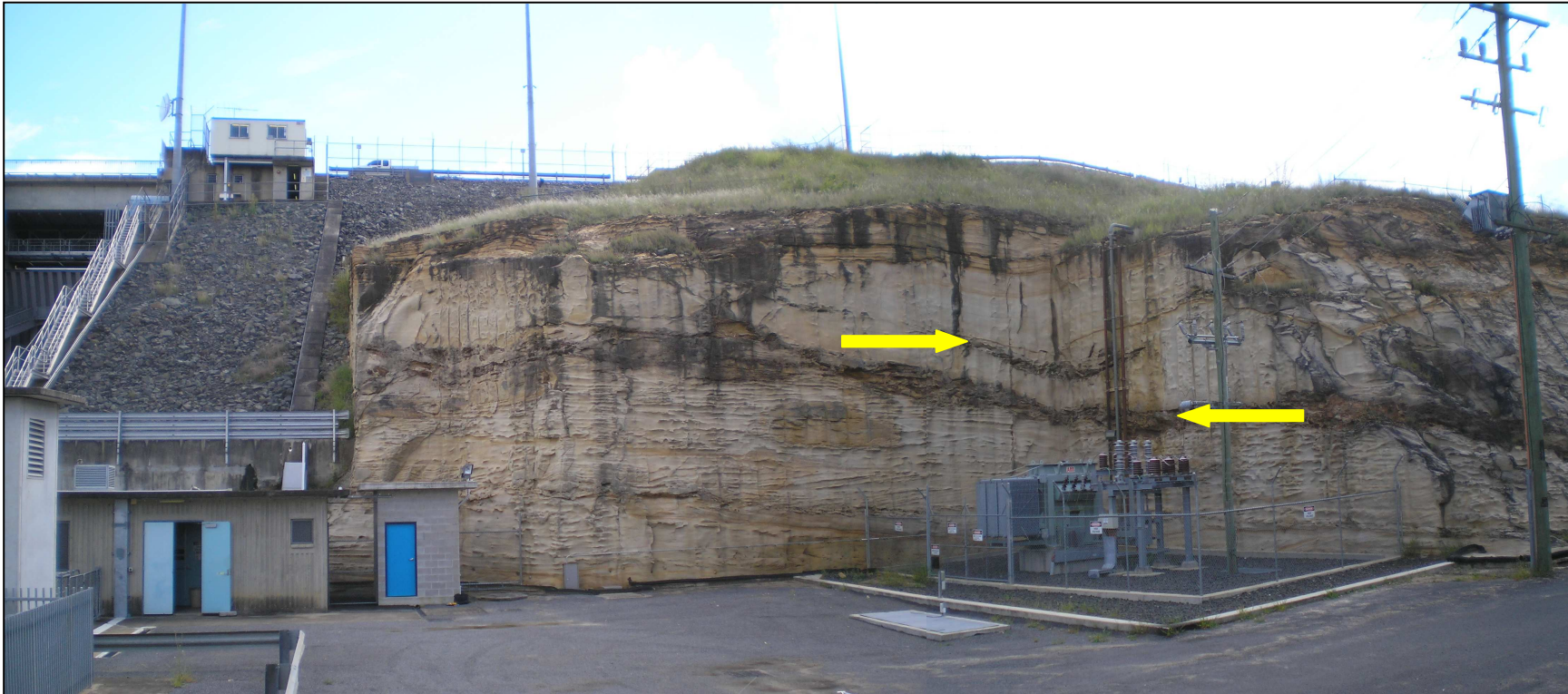
Photo 1: View of cutting looking towards north. Electrical substation located to right and workshop buildings located to left. Highly weathered siltstone beds arrowed.
