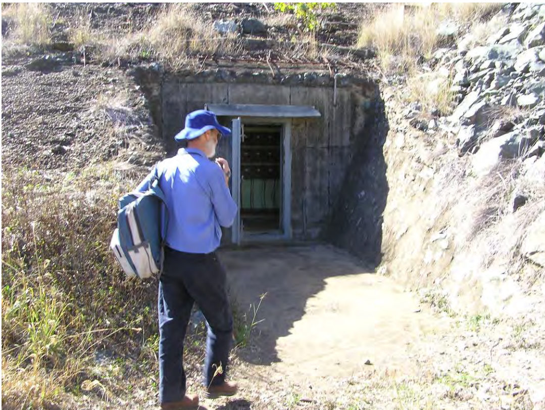
Photograph No. 16: Instrumentation Terminal Structure at Toe of Right Embankment
