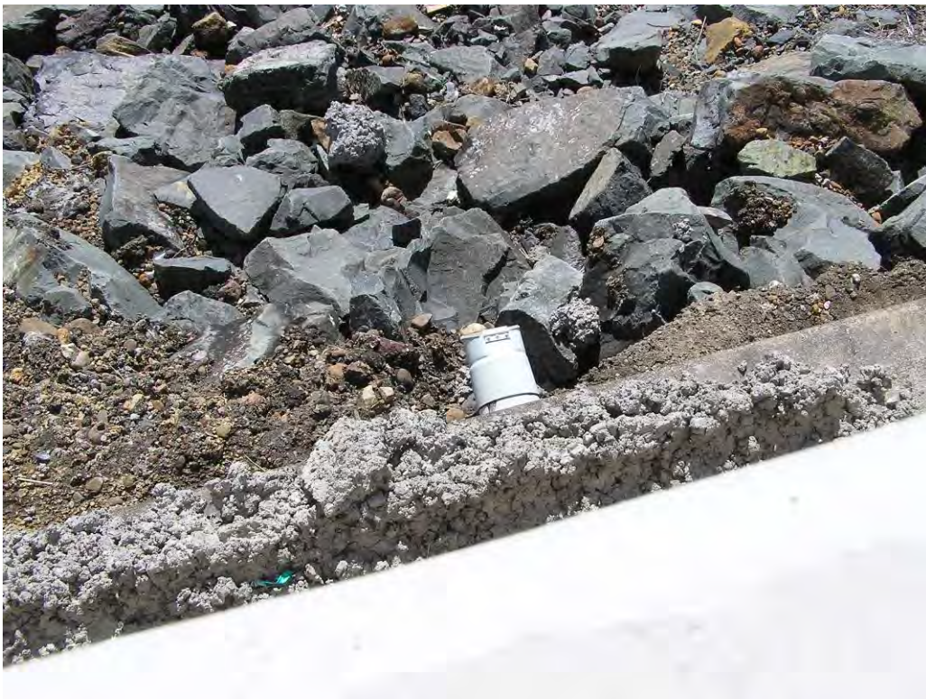
Photograph No. 8: Main Embankment - Road Drains Discharging to U/S Side Showing Flap Valves
