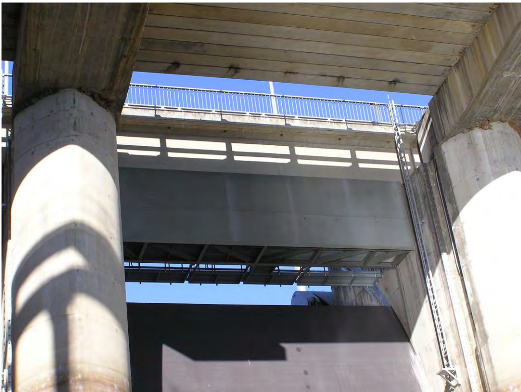
Photograph No. 2: New Baffle Structure Above and U/S of Radial Gate
