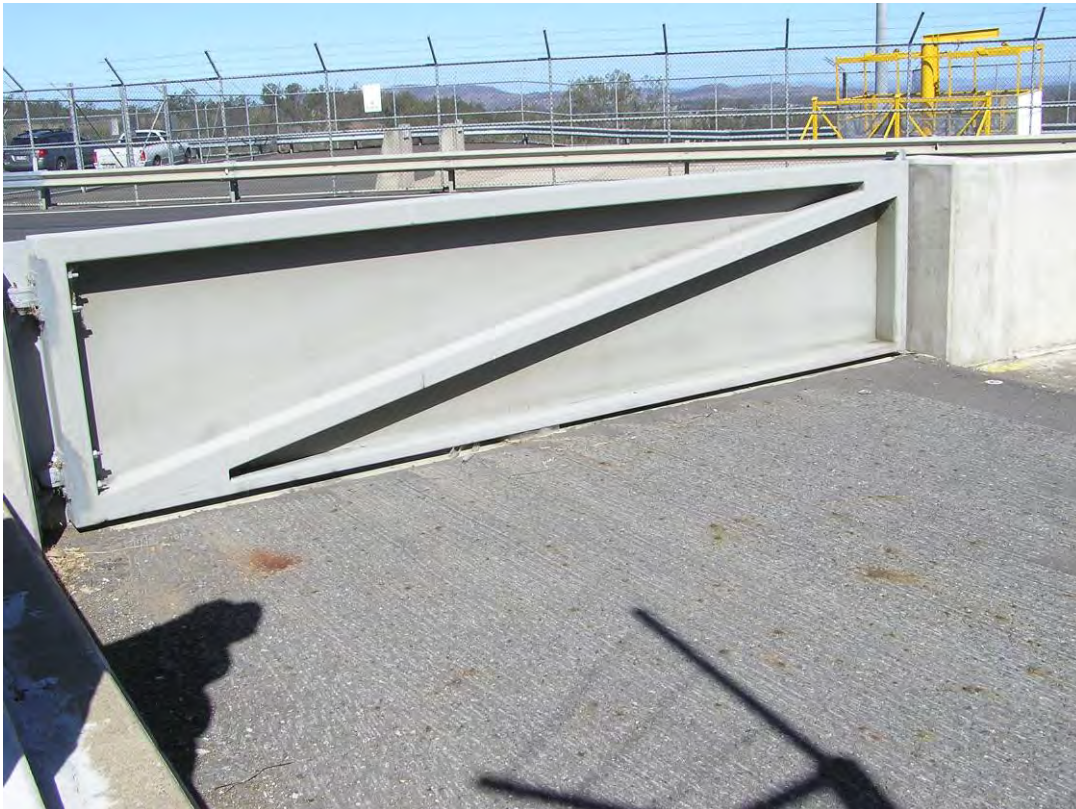
Photograph No. 10: "Watertight" Gate Adjacent to Spillway - Requires Rubber Seals
