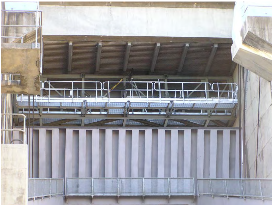
Photograph No. 18: New Spillway Baffle From D/S
