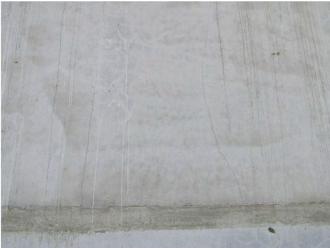
Photograph No. 4: Auxilliary Spillway Left Hand Inlet Training Wall Showing Cracking
