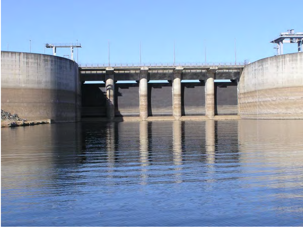
Photograph No. 1: U/S of Spillway Showing Radial Gates
