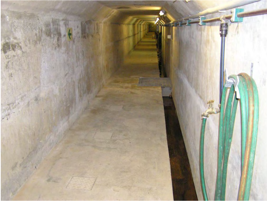
Photograph No. 19: Gallery Inside Spillway Crest
