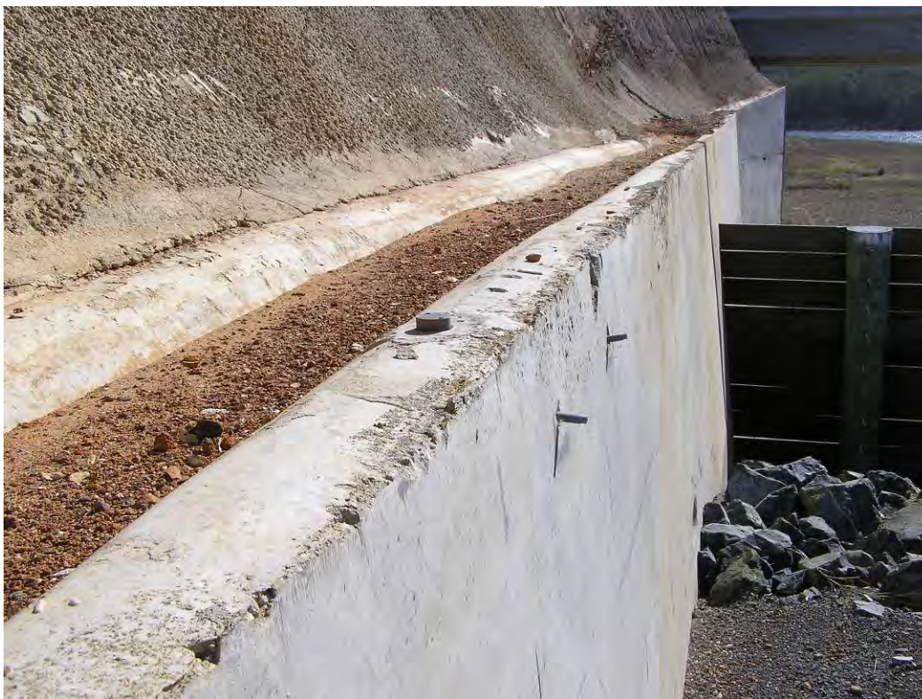
Photograph No. 5: Right Hand Auxilliary Spillway Abutment Wall Showing Debris Filled Gutter
