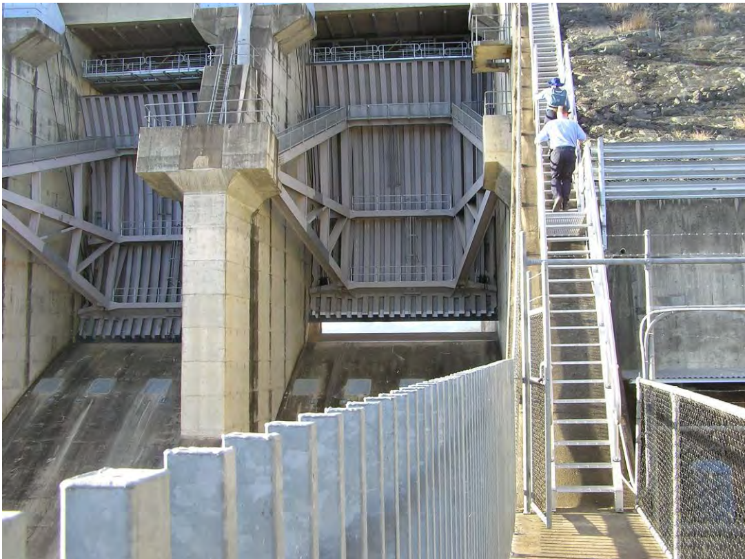
Photograph No. 20: No. 1 Radial Gate Being Raised
