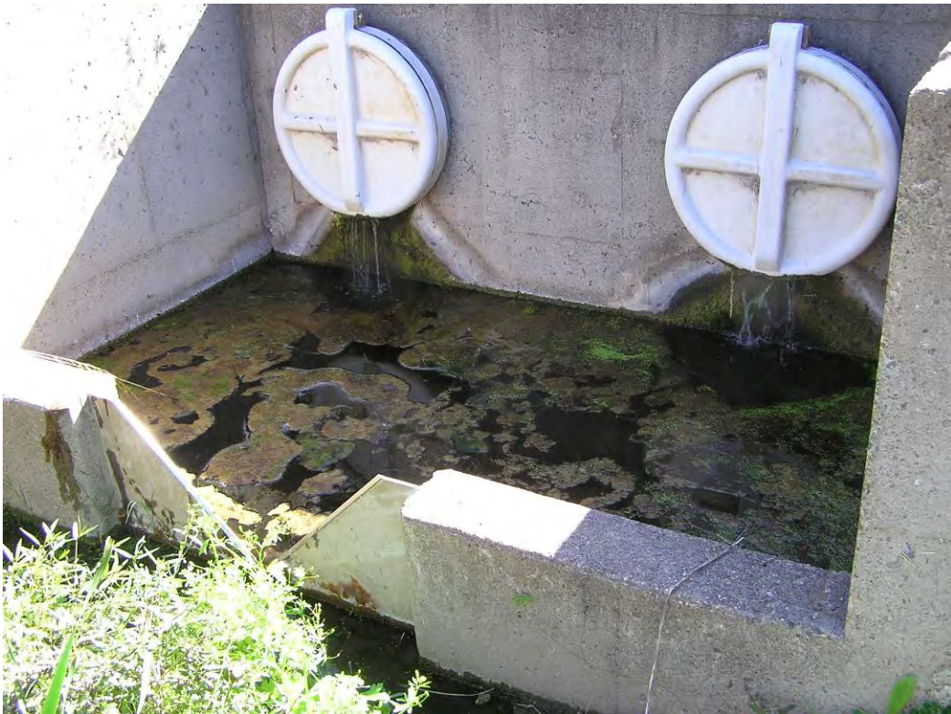
Photograph No. 14: Drainage/Seepage Collection D/S of Right Embankment
