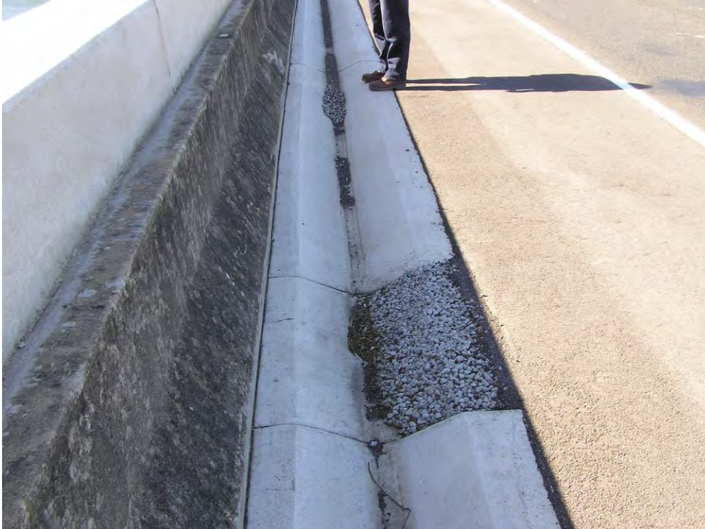
Photograph No. 9: Main Embankment U/S Road Drain Showing 'No-fines Concrete' Around Drainage Discharge Point
