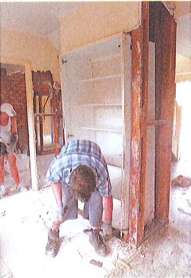
removing kitchen pantry
