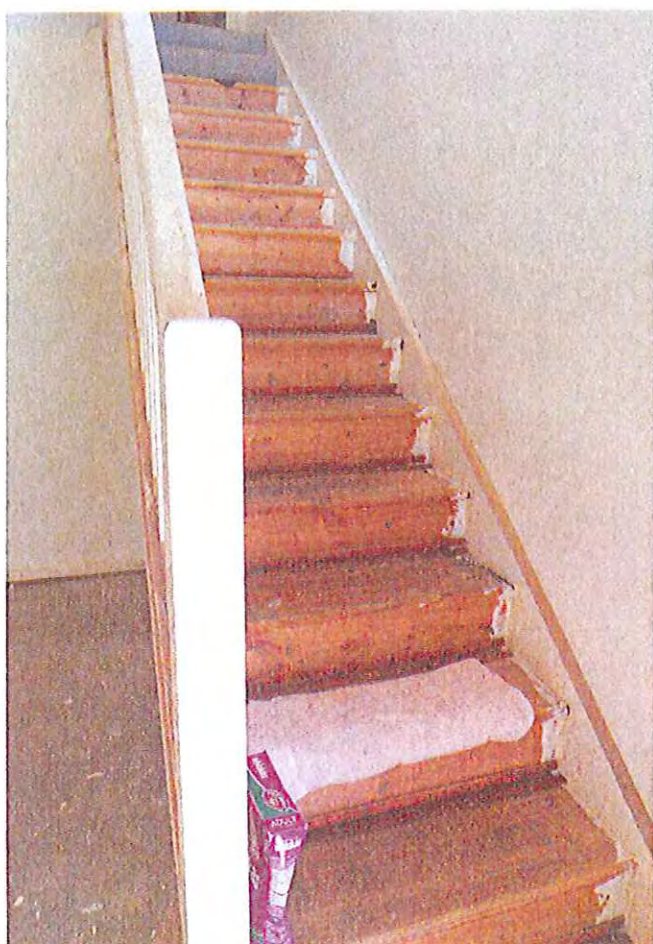
o carpet from stairs removed
