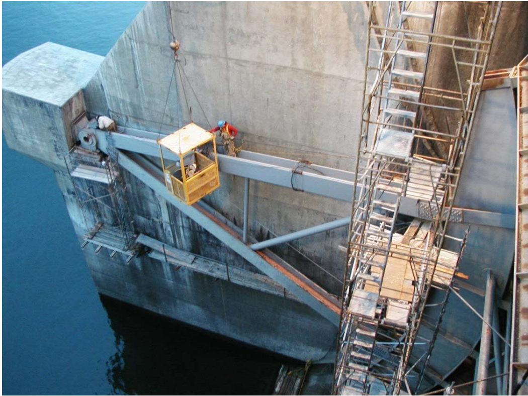
Photo 3 Priest Rapids Dam Washington State USA
