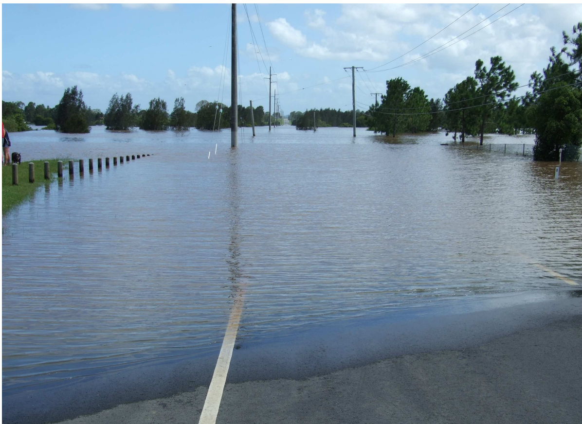
Figure 4 – Existing Loganlea to Jimboomba (F820) 110kV powerline with 1.2 kms of Logan Reserve Road flooded and restricting access during the January 2011 Logan River flood.
