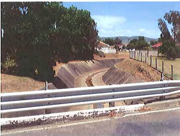
Coming From "The Basin" Concrete lined creek coming into Cessnock.
