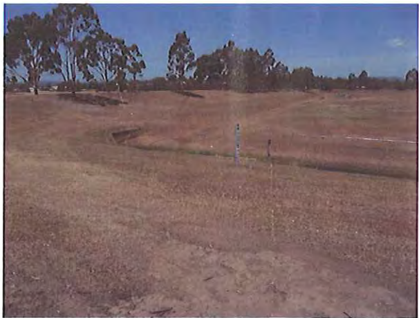
The Exit Outlet Pipe area. Note the two Water Depth Markers. The Left Marker measures 2-4 meter deep water. The Right Marker measures 0-2 meter deep water.
