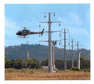
The major program of work under way to reinforce supply to north Mackay saw the construction of a new bulk supply substation at Glenella in Mackay during the past year, along with a major powerline from Pioneer Valley to Glenella, shown here with the line being strung by helicopter. The final stage, one of the many projects now under way as part of the delivery of this year Network Management Plan, is a new feeder from Glenella to the existing north Mackay zone substation.
