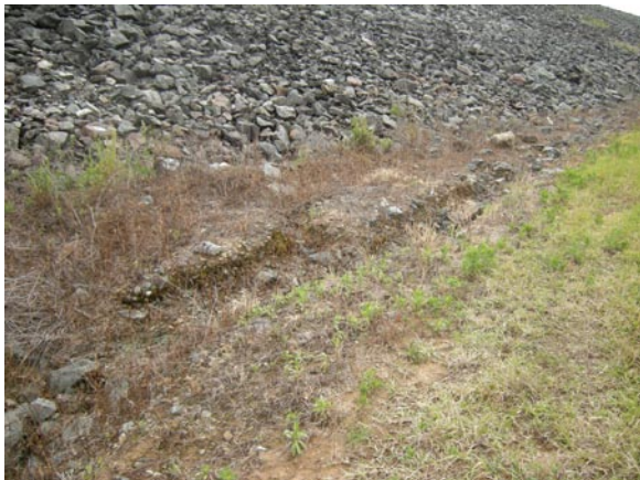
Erosion areas to be repaired along toe
