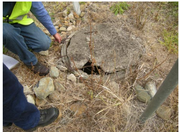
Broken inspection pit cover
