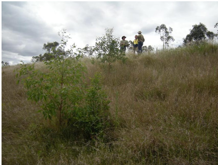
Trees on Saddle Dams to be removed
