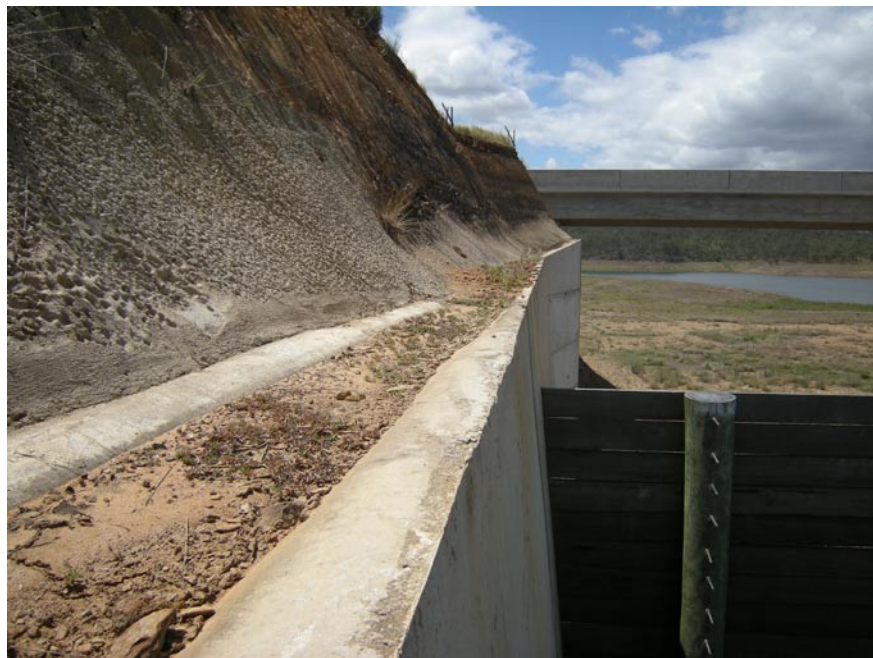
Drain to be cleaned
