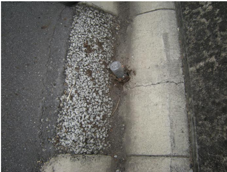
Broken/Blocked Road Drain
