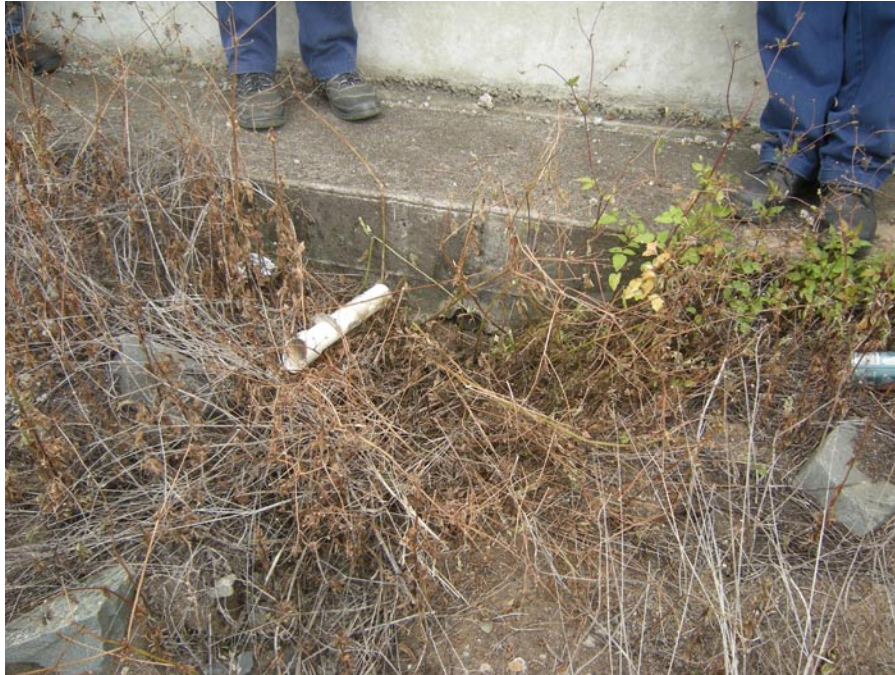
Broken/Blocked Road Drain
