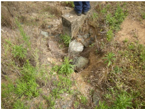
Erosion areas to be repaired along toe
