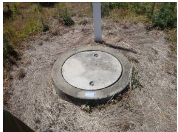
Repaired Pit and new Marker Post
