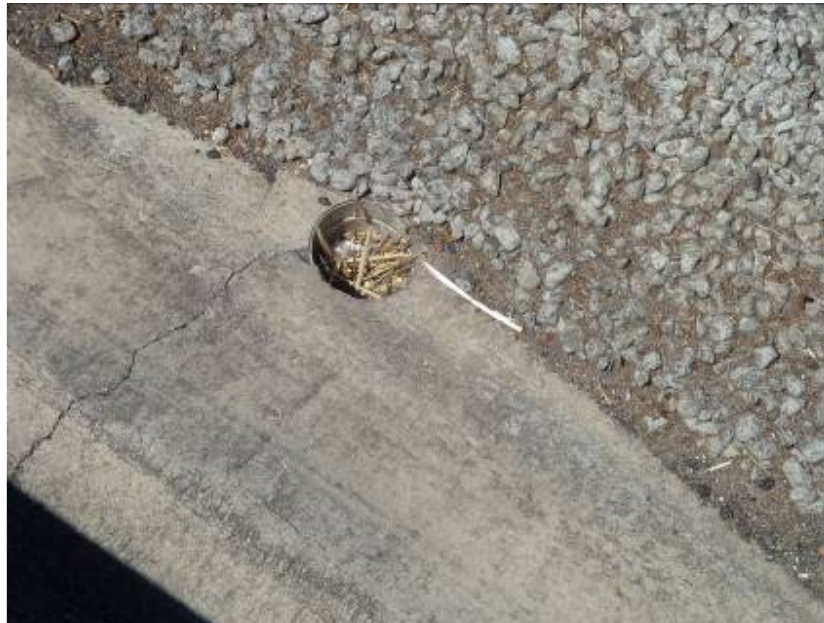
Broken/Blocked Road Drain
