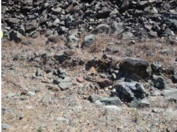
Minor erosion areas to be repaired along toe
