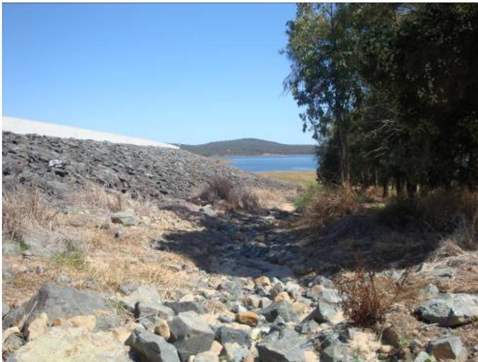
Left Bank Embankment – Trees to be removed
