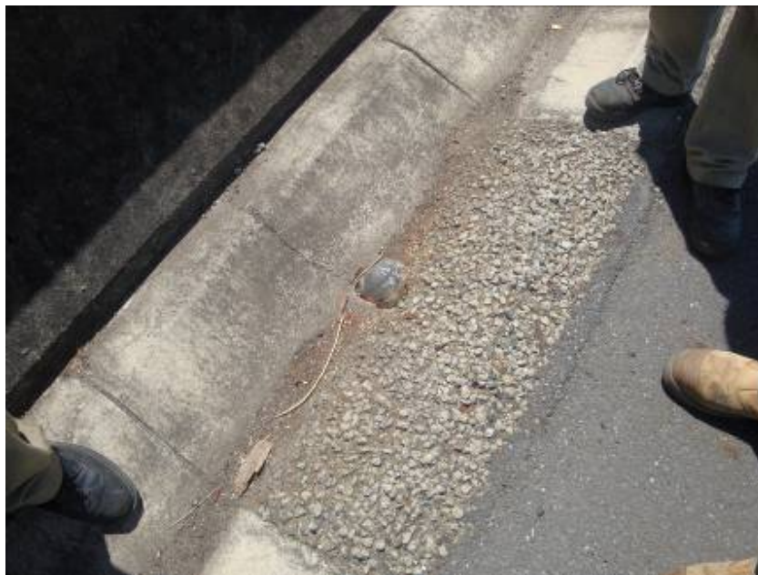
Broken/Blocked Road Drain
