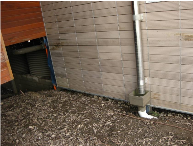
Figure: View on eastern side of entrance showing the water line
