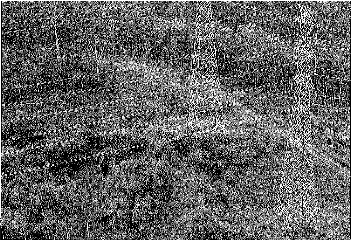
Figure 3 - Landslip near tower at Mt England
