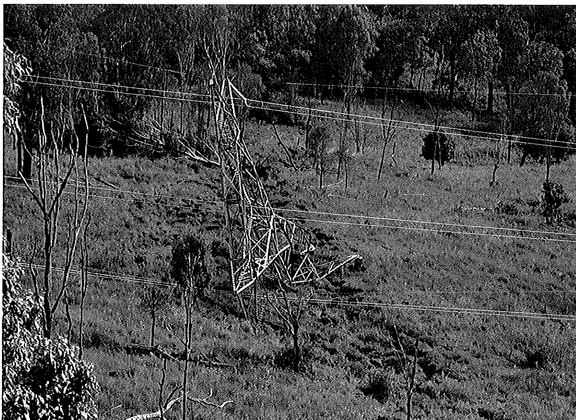
Figure 1 - Landslip damages tower on feeder 832
