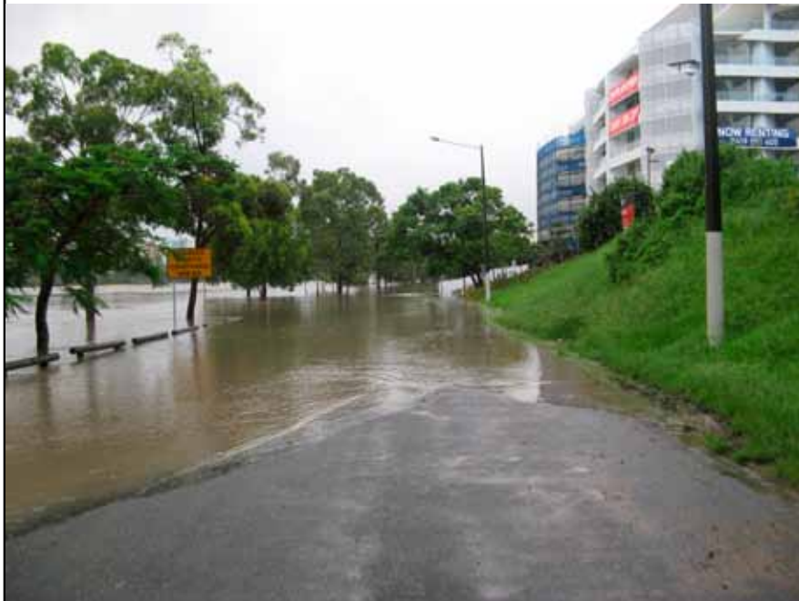
View of Riverside Drive at 6.33 pm on 11/01/11 showing Waters Edge on the right
