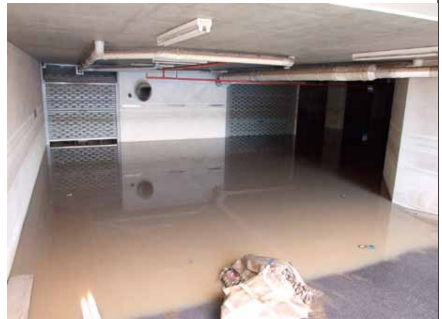
Aura carpark entrance showing room where pool controls are housed in room (left) on Basement 1
