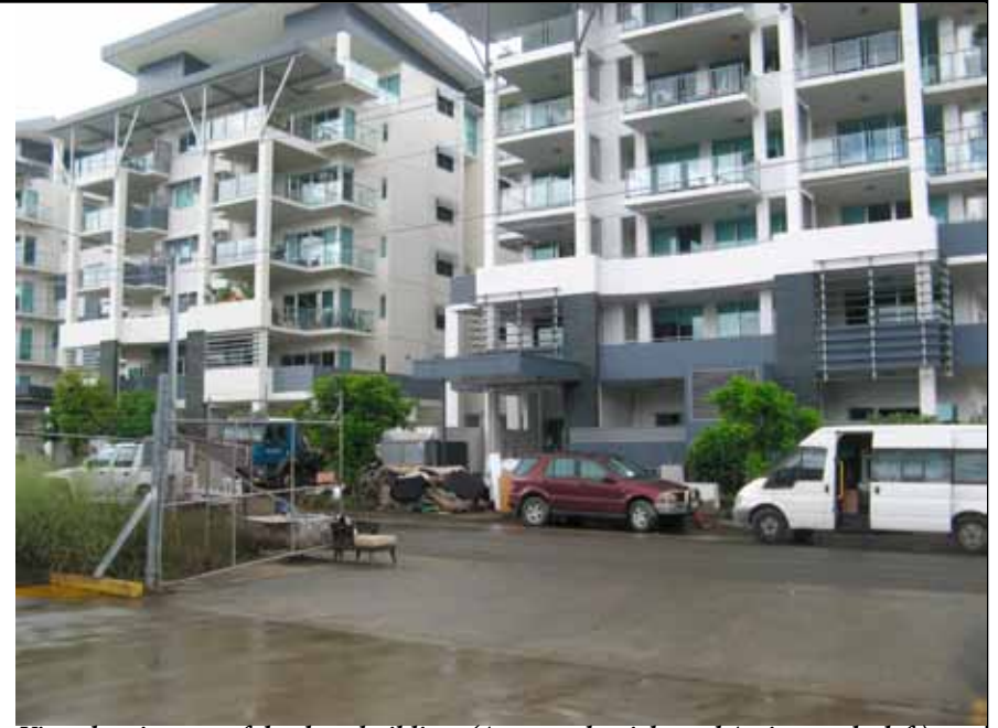
View showing two of the three buildings (Aura on the right and Arriva on the left) serviced by the Energex transformers
