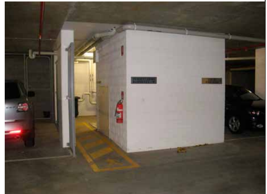
Lift well in Aura in Basement 2 with the main lift motor behind the yellow door in the wall near the fire extinguisher
