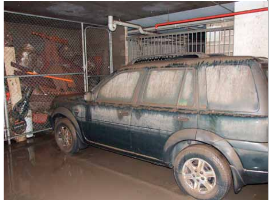
Car and contents submerged in Aura basement
