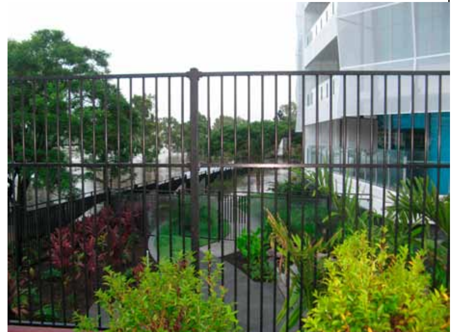
View of water entering Waters Edge on 12/01/11 at 5.08 am
