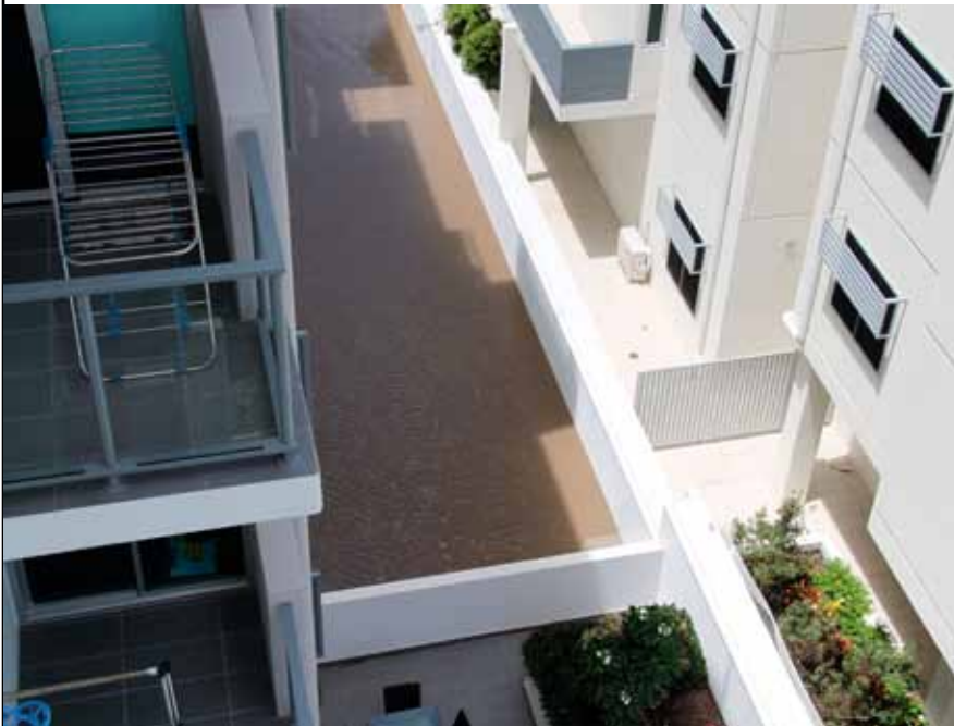
View of the carpark entrance with water still rising at 1.19 pm on 12/01/11
