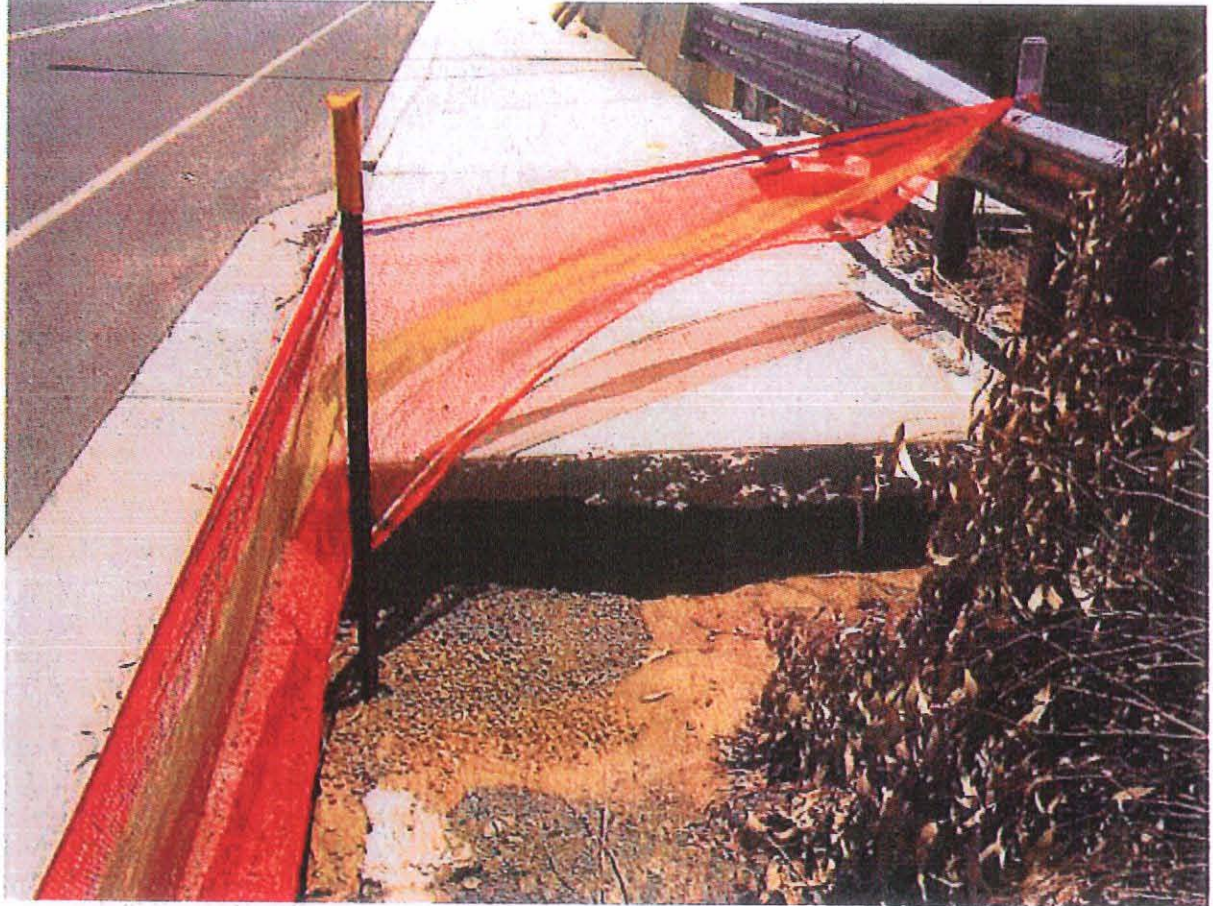
1. Three Mile Bridge - Erosion
