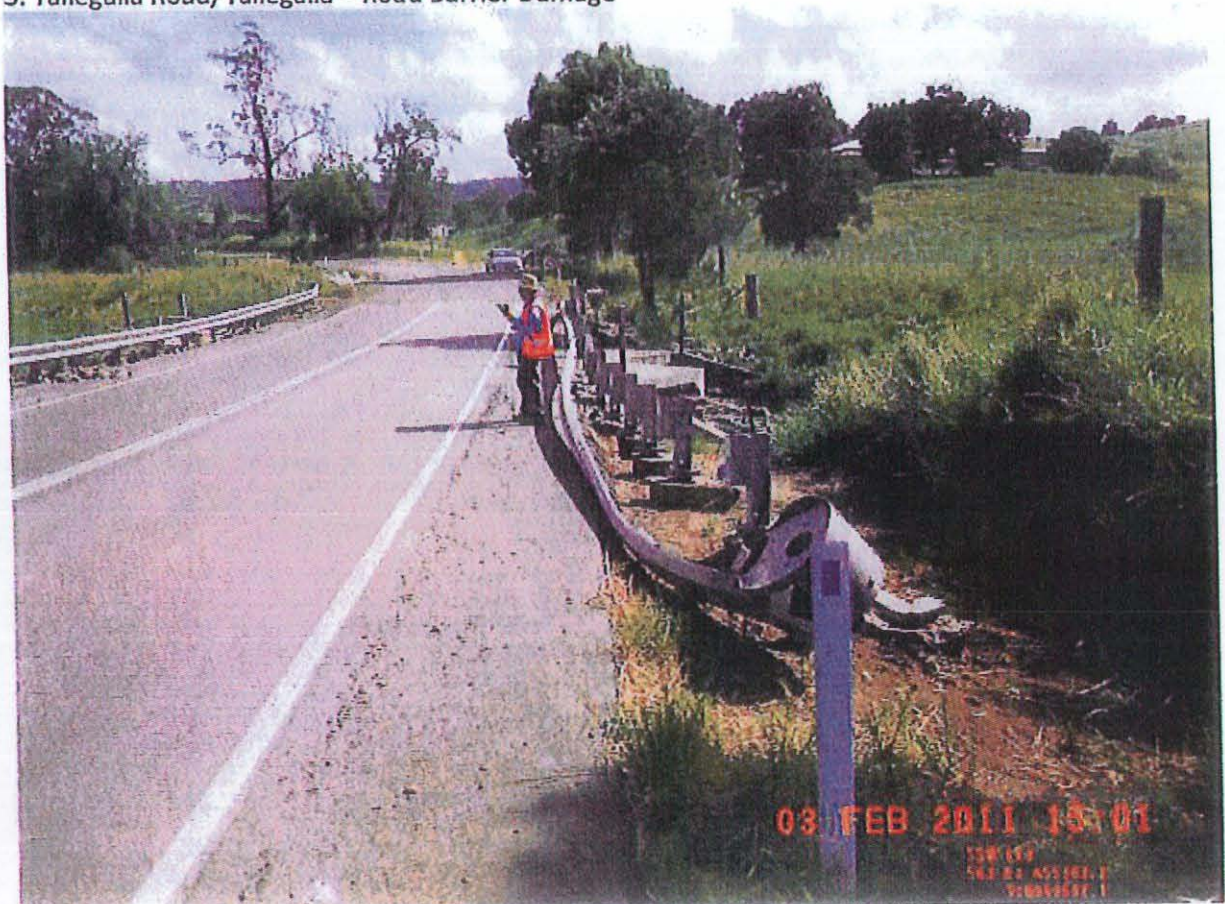
3. Tallegalla Road, Tallegalla – Road Barrier Damage
