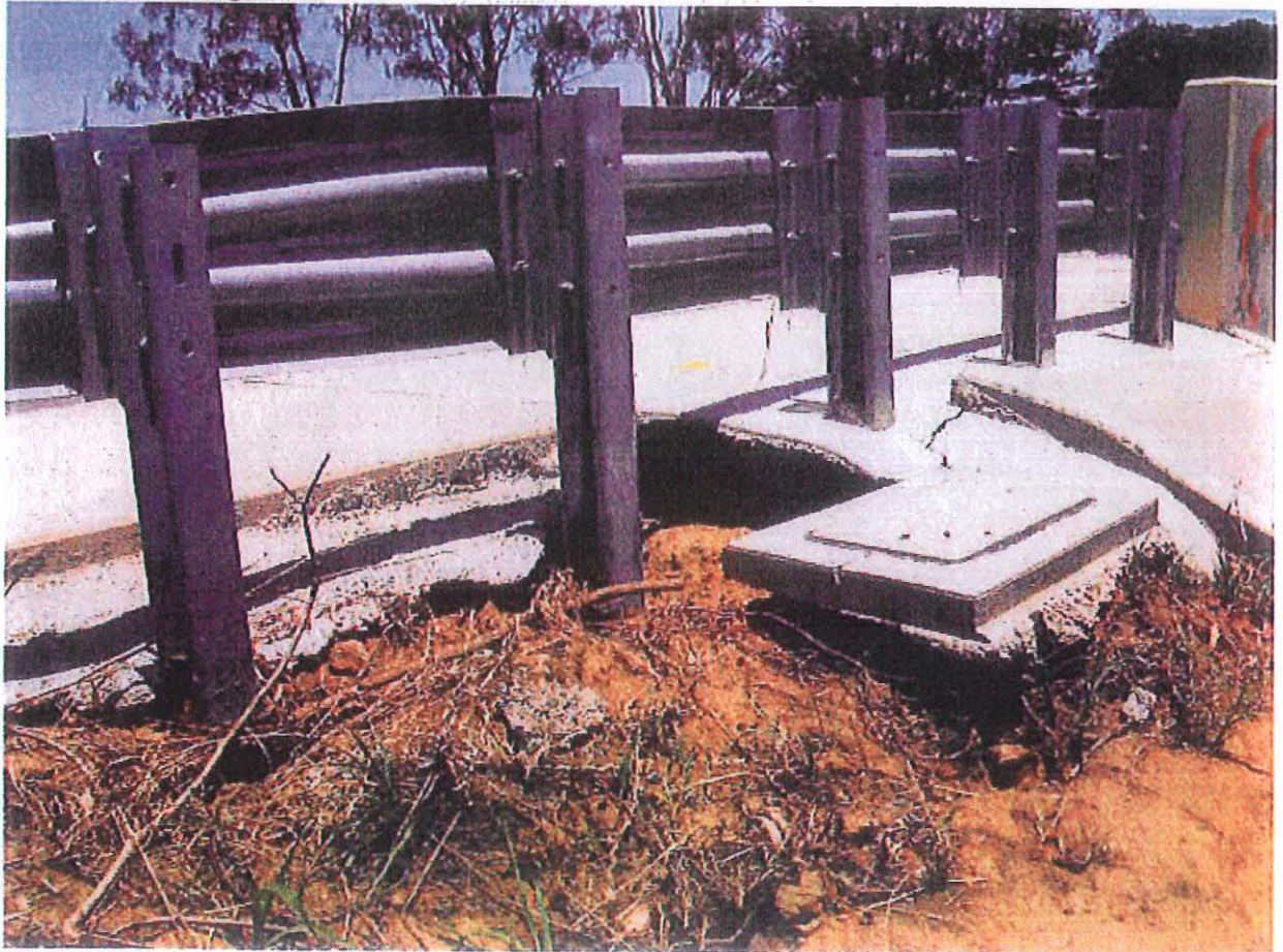
1. Three Mile Bridge - Erosion
