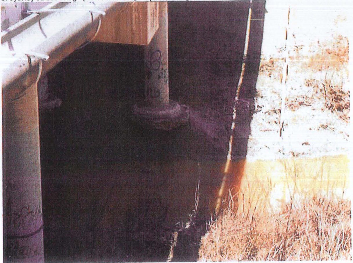
5. Sydney Street Bridge (Iron Pot Creek) – Erosion
