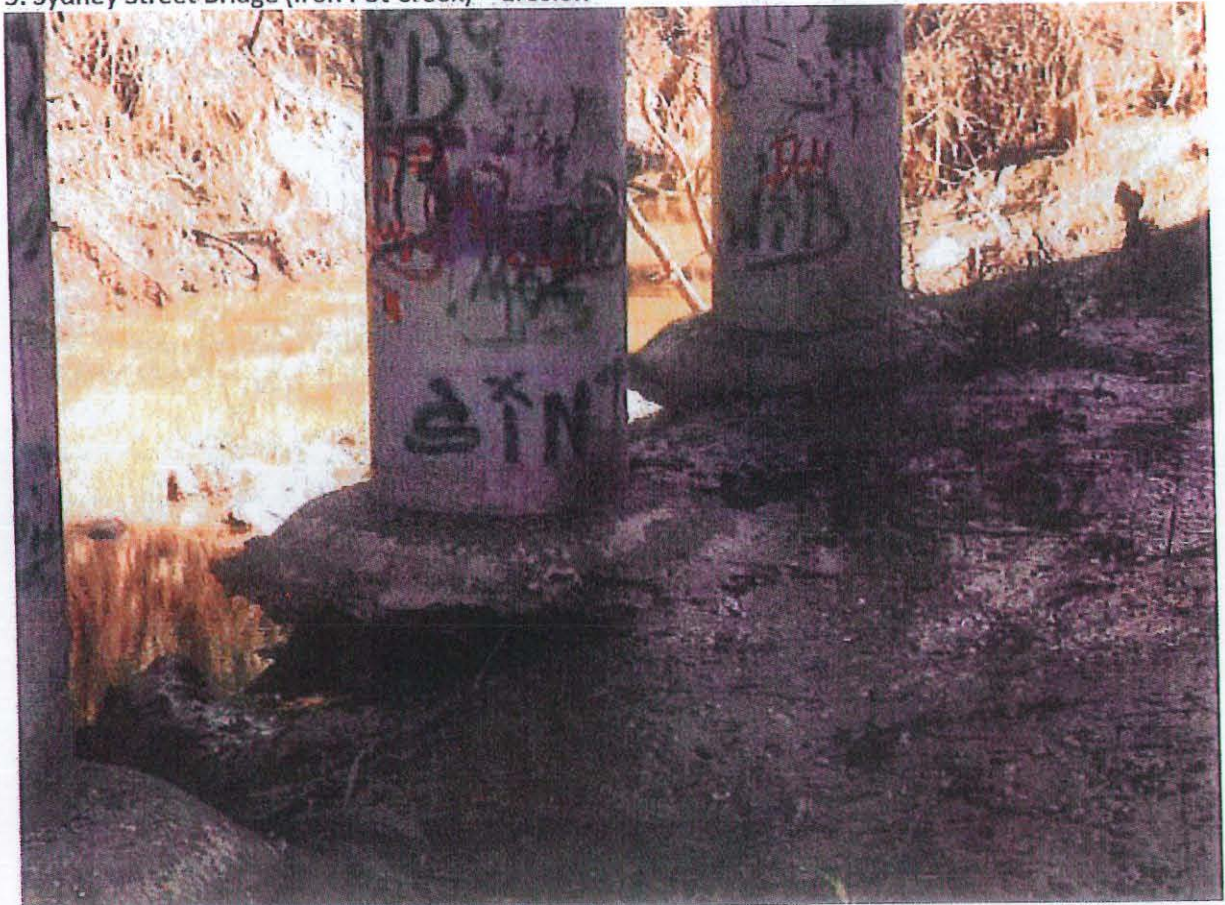
5. Sydney Street Bridge (Iron Pot Creek) – Erosion
