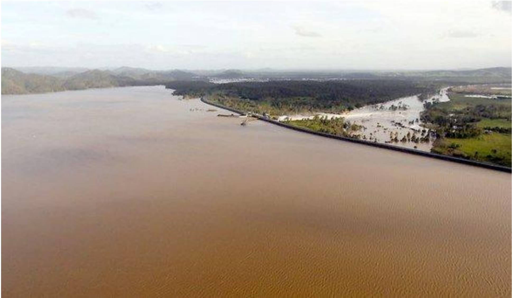
Figure 11: Wivenhoe on Wednesday 12 January 2011 at 8:46 am: Imagine the wall over-topping and eroding, and the Lake bursting downstream: A Dam-Burst-Tsunami-Flood-Wave
