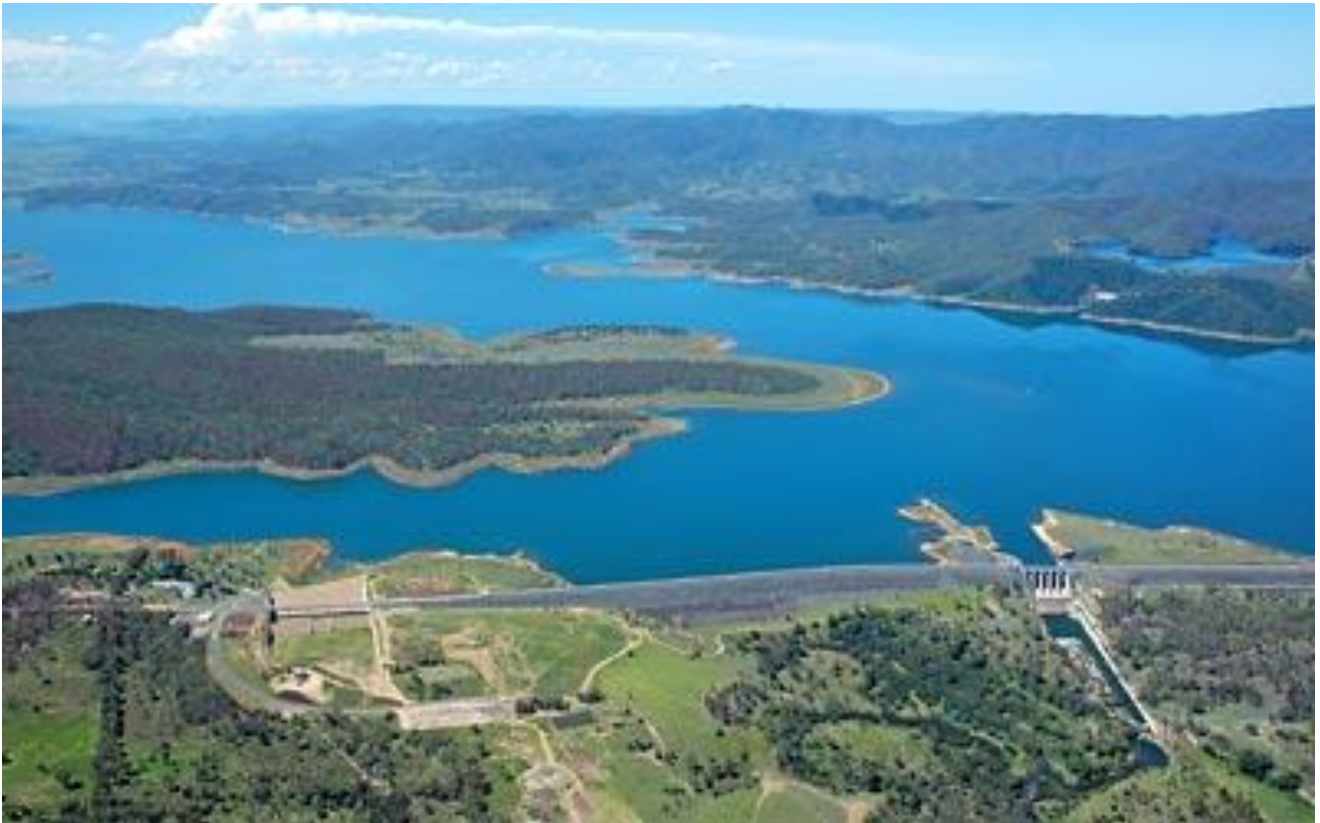
Figure 1: Wivenhoe Dam with Fuse Plugs at left and gates at right.
