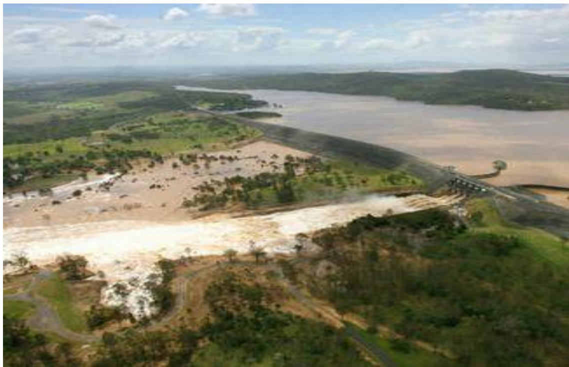
Figure 4: Wivenhoe in January 2011. The gates are at the right, and the fuse plugs near the top centre of picture
