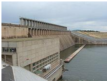
Figure 33: The Hume Weir's concrete gates in the foreground, and the earthen wall in the distance
