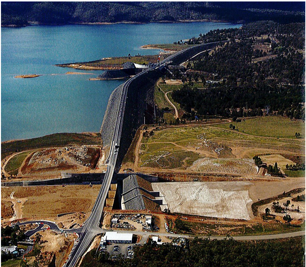
Figure 7: The Wivenhoe Fuse Plugs prior to the 2011 flood
