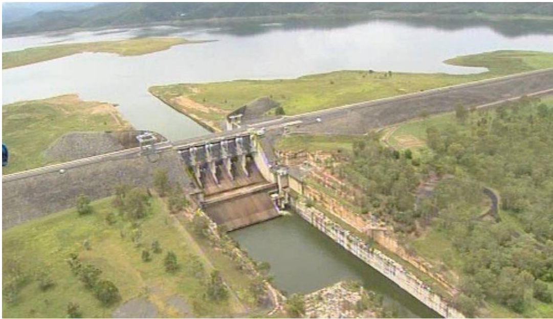
Figure 37: The extent of the rock can be seen near the Wivenhoe gates
