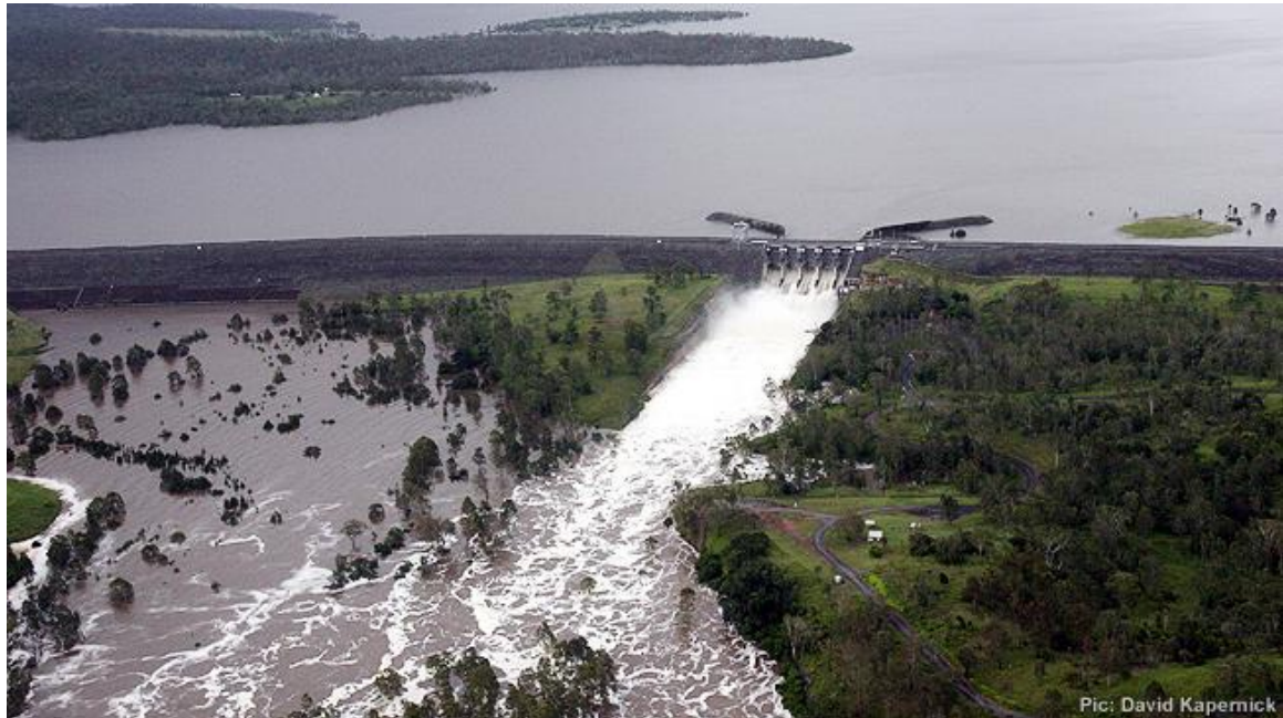
Figure 3: Wivenhoe dangerously full on Monday 10 January 2011
