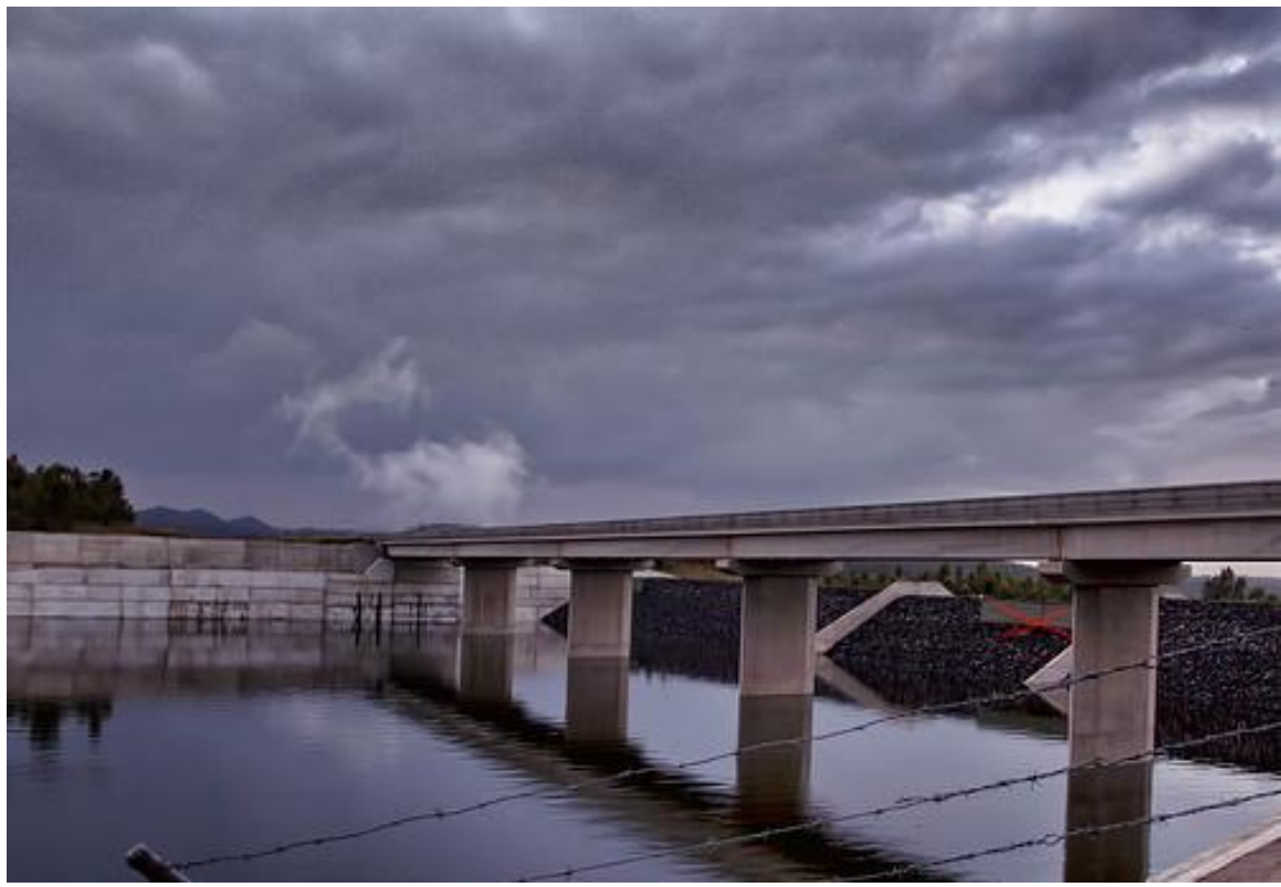
Figure 9: Fuse plugs with water on the way down. See the high water mark on the pillars of the Brisbane Valley Highway.
