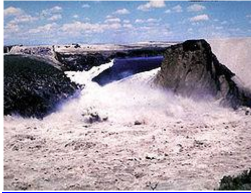
Figure14: The collapsing Teton Dam
