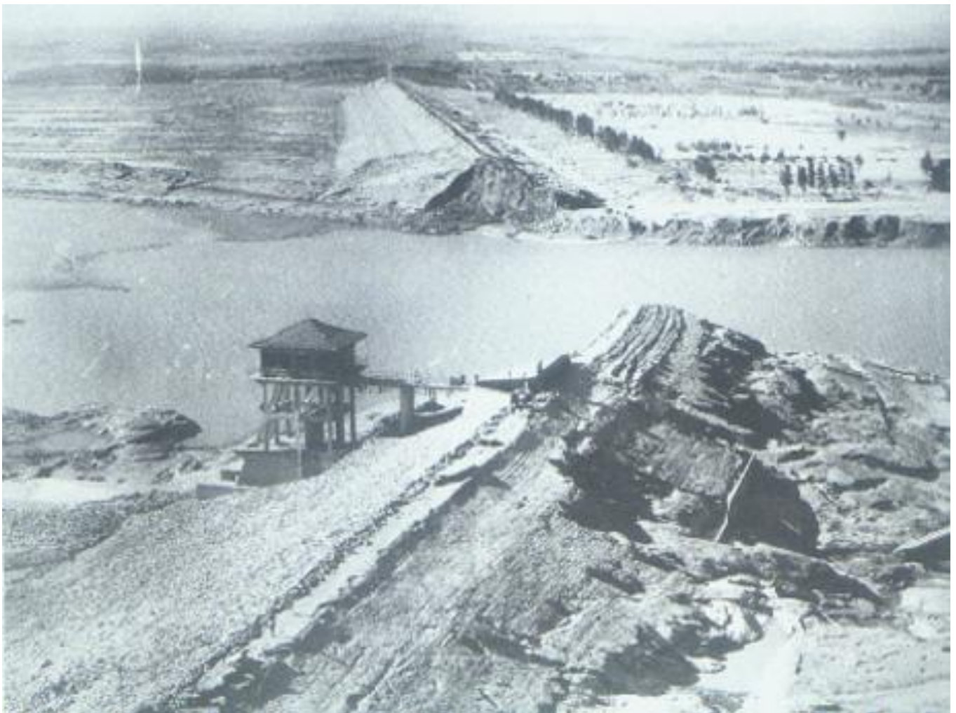
Figure 12: The collapsed Banqiao Dam after flood-water over-topped and eroded the earthen wall
