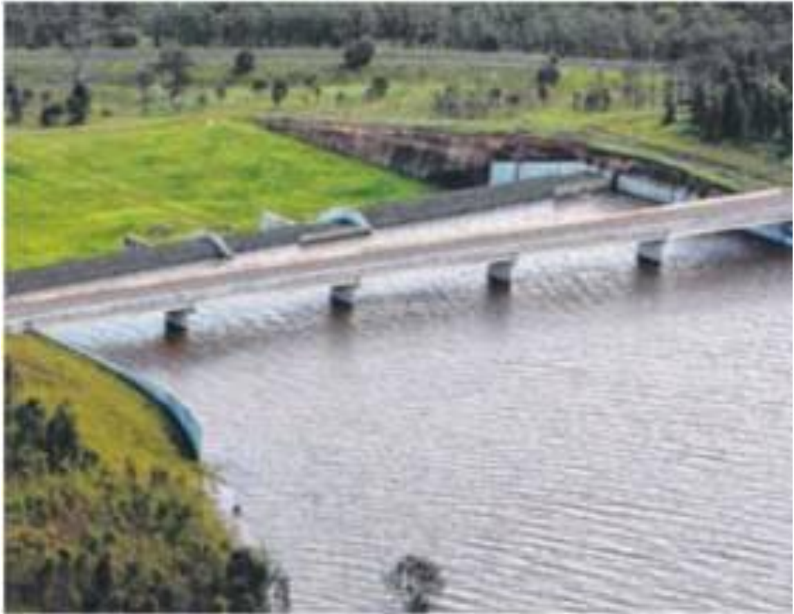
Figure 8: The Wivenhoe Fuse Plugs getting close to over-topping
